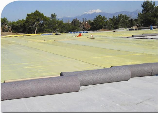
Geo-textile without mesh is the name of the product by means of which those synthetic short fibres are combined mechanically by method of needle. There is no warp or weft in geo-textile without mesh. On the other hand, its endurance is ensured by means of heat treatment and the intermingling of fibres.
