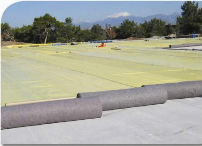
Geo-textile without mesh is the name of the product by means of which those synthetic short fibres are combined mechanically by method of needle. There is no warp or weft in geo-textile without mesh. On the other hand, its endurance is ensured by means of heat treatment and the intermingling of fibres.
